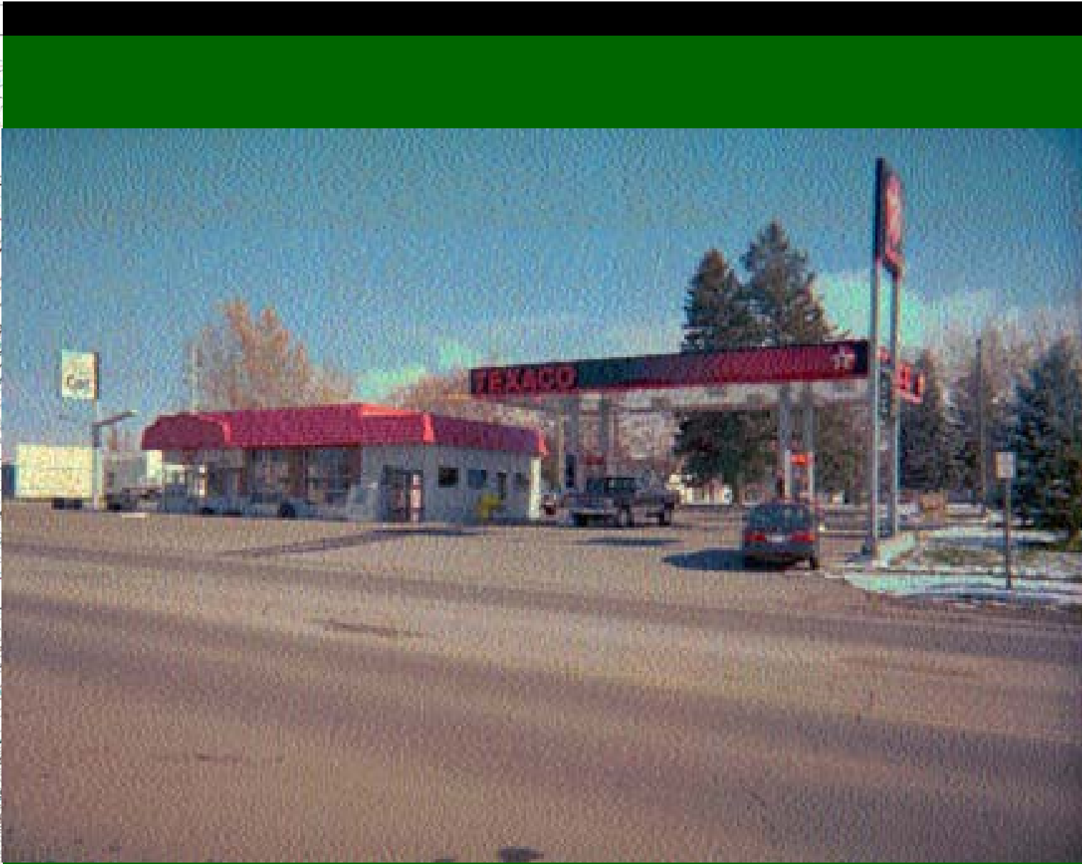
Site J – Randy's Texaco, View to NE
